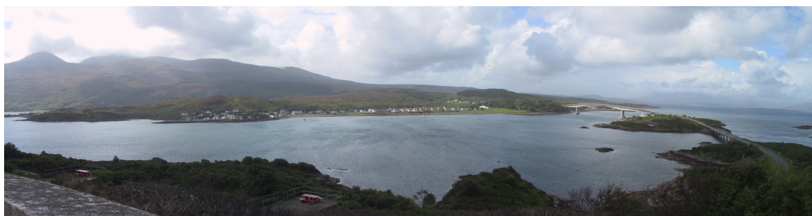
Kyleakin (Skye), Loch Alsh and the Skye bridge (right) taken 2004.
